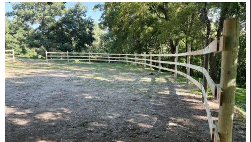
New arena fence
